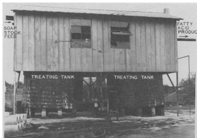
FIG. 2. Front view of soap stock conversion plant.
